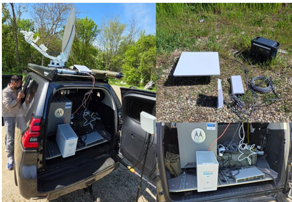
Figure 76 : Equipment installation on the emergency intervention car
