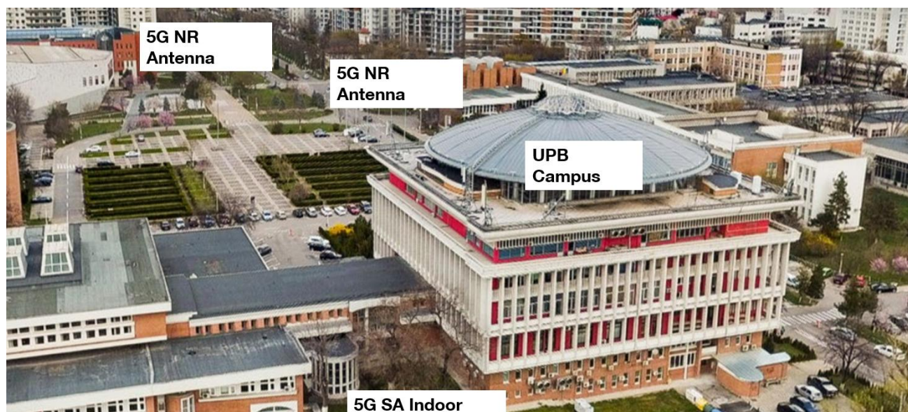
Figure 30. Private 5G SA infrastructure deployed at the UPB Campus in Bucharest.
